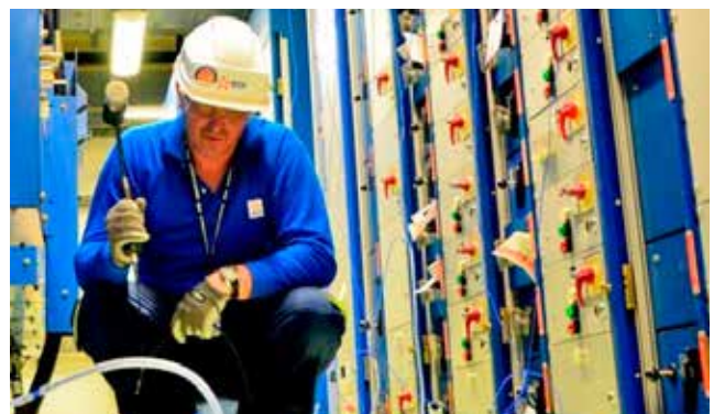
Tests on electrical cubicles
