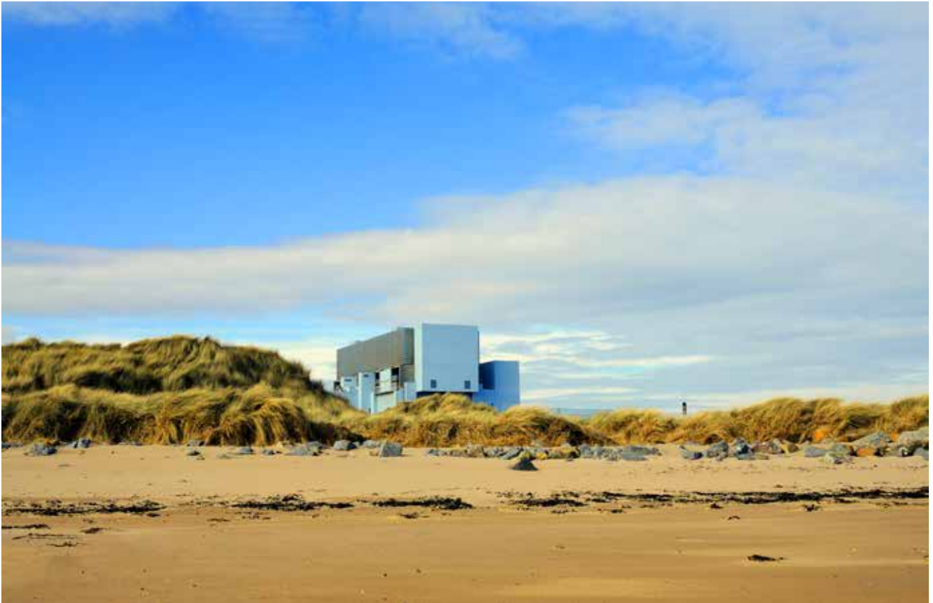
Torness nuclear power plant
