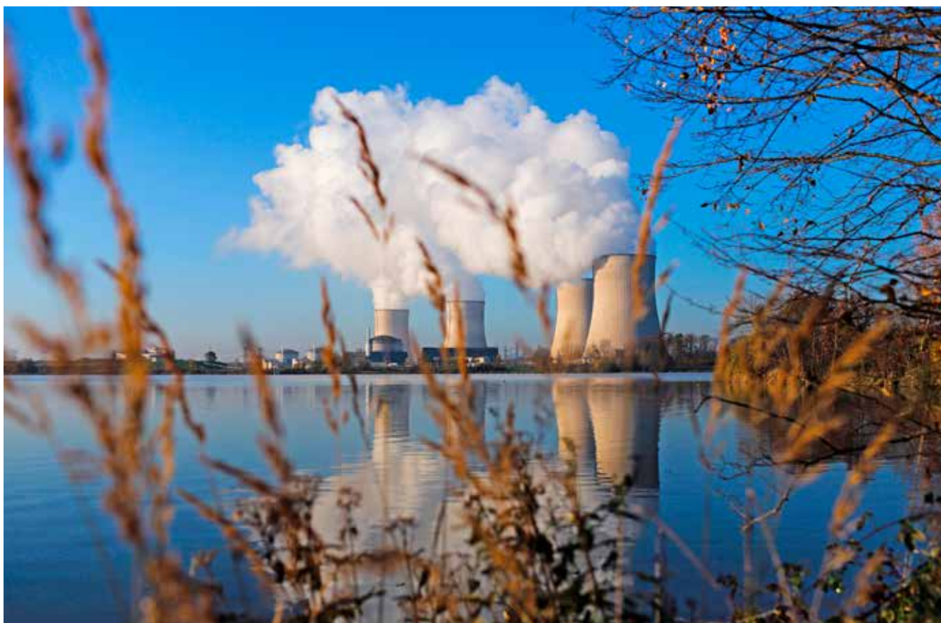
Cattenom nuclear power plant
