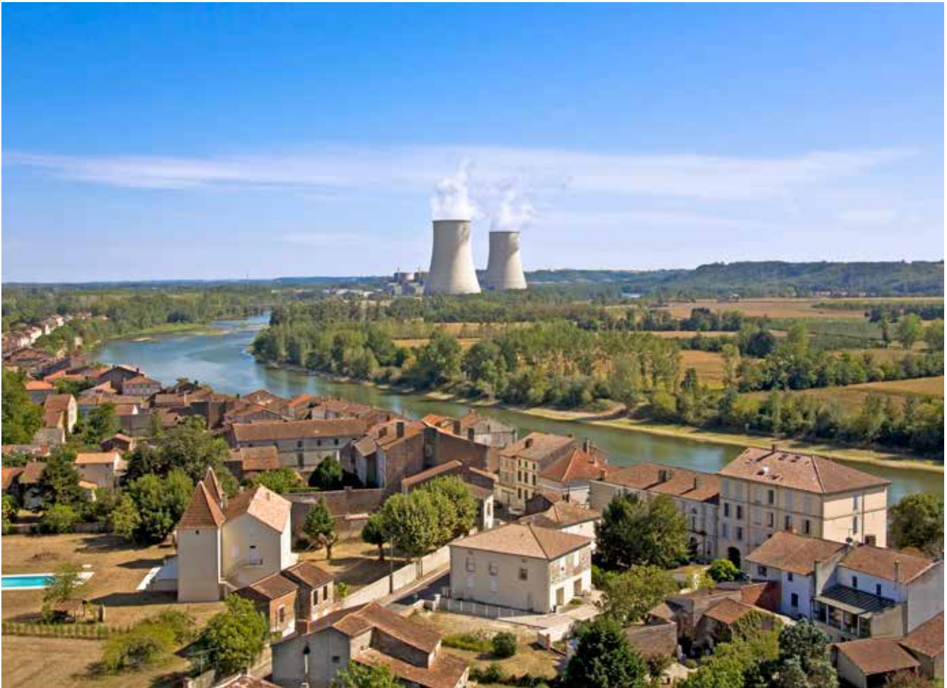
Golfech nuclear power plant
