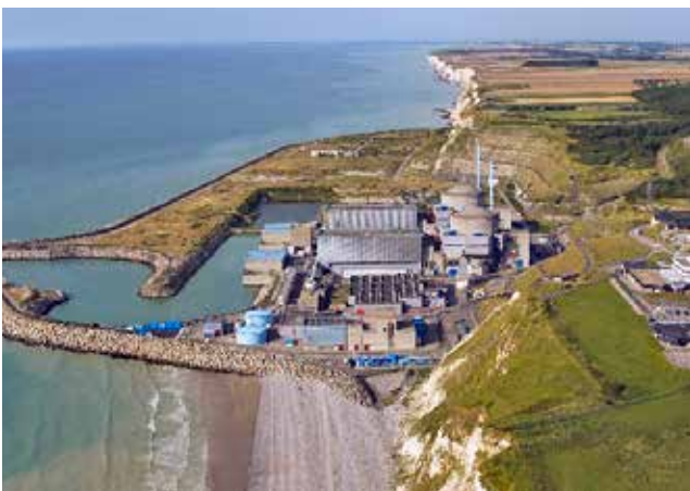
Penly nuclear power plant
