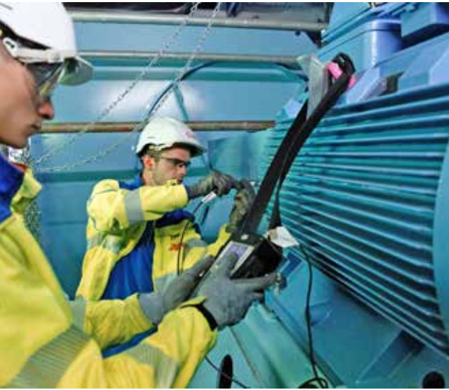
Assembly operations on the Flamanville 3 site
