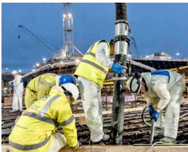
HPC construction site
