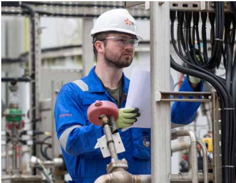
Maintenance activity, Hinkley Point B
