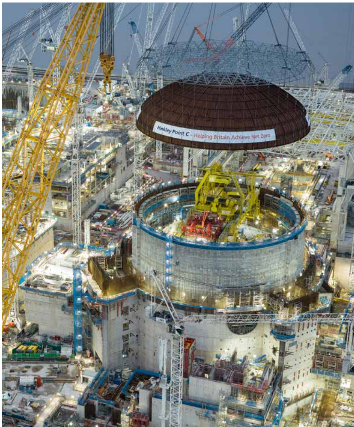
Placing HPC Reactor 1 dome
