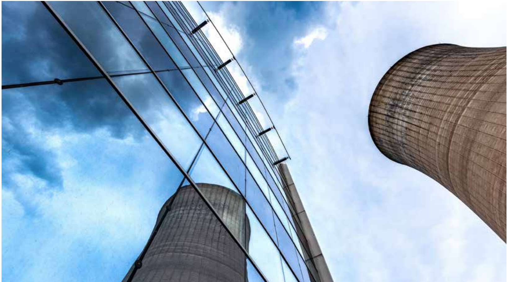
Dampierre-en-Burly power station
