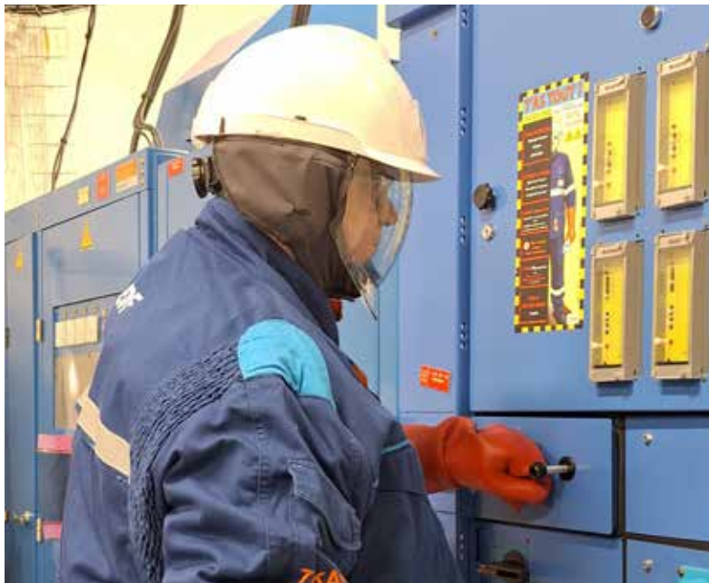
Operations in an electrical cubicle, Saint-Laurent-des-Eaux B
