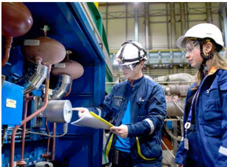
A C&I activity in the turbine hall, Flamanville 1&2
