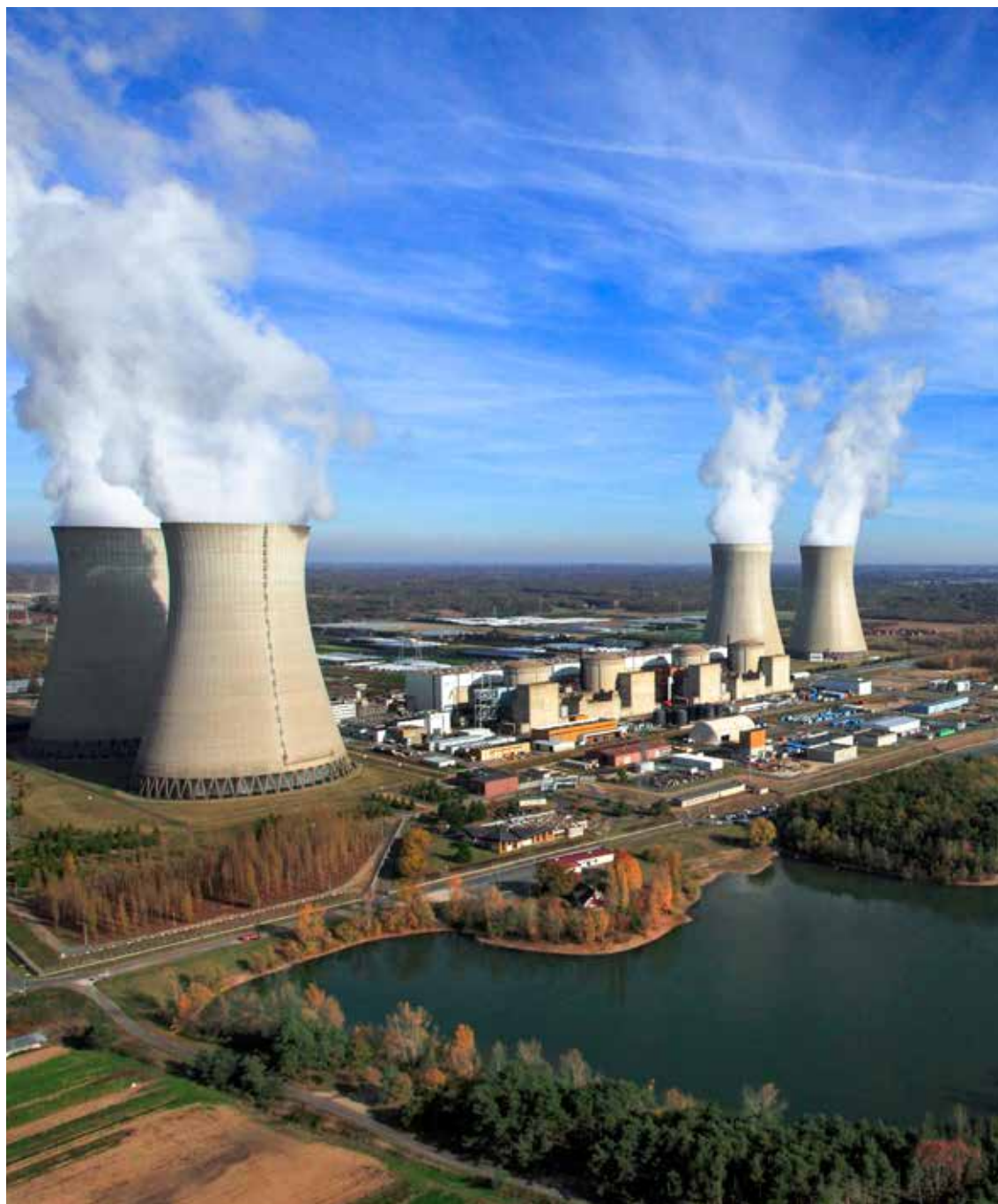
Dampierre-en-Burly power station
