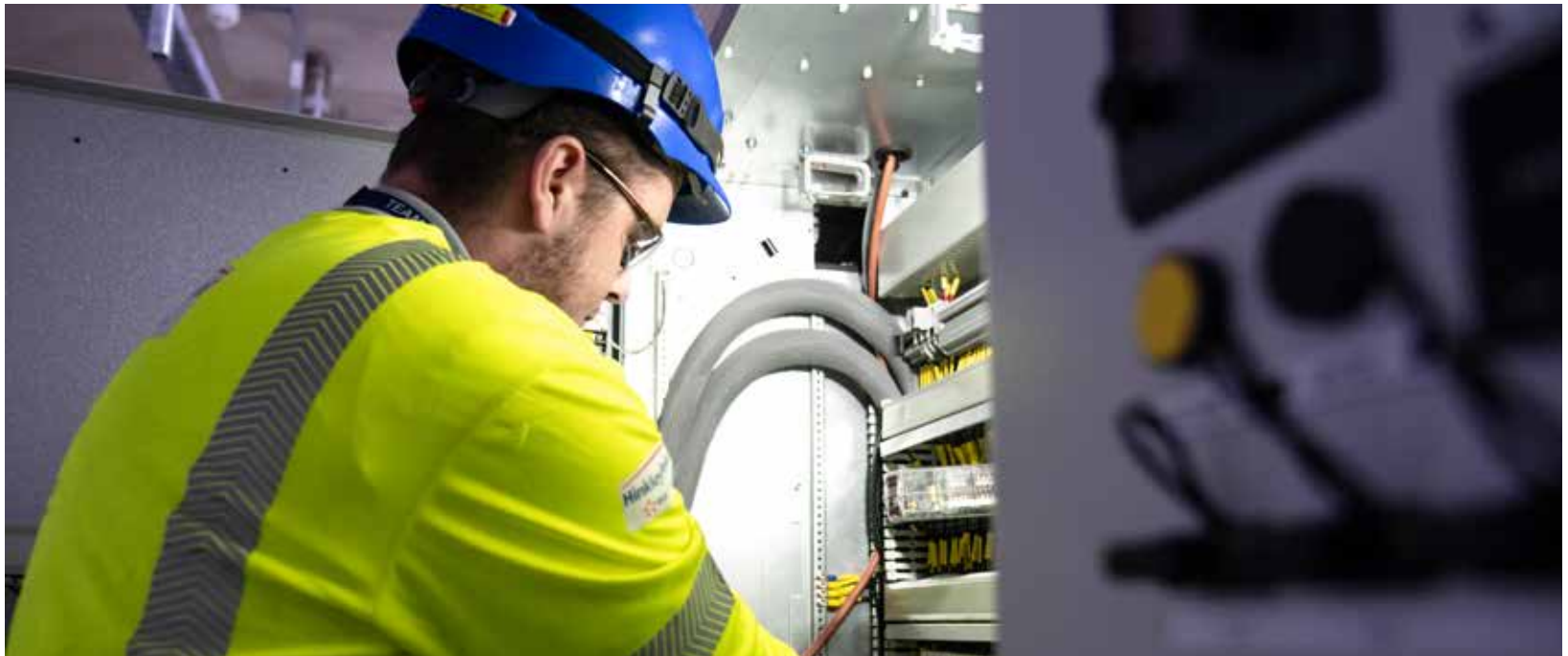
Electrical installation activity, HPC
