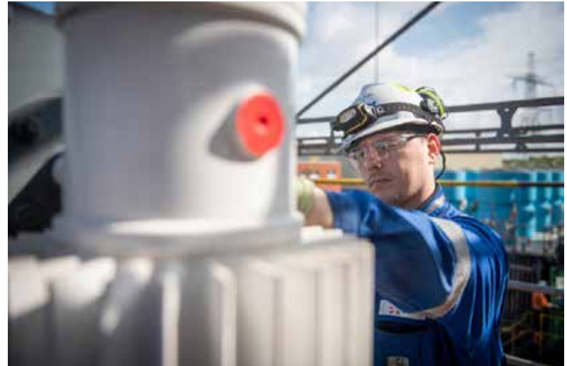
Transformer inspection, Heysham 2
