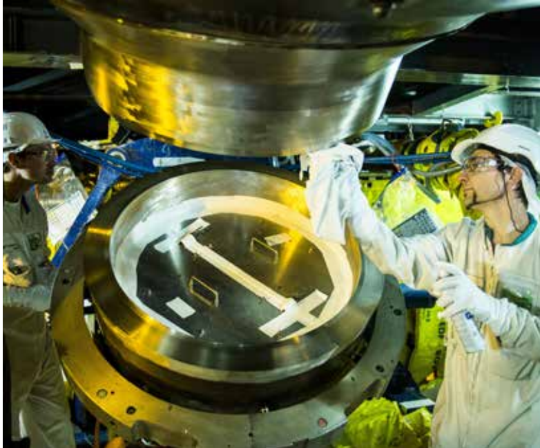
Steam generator replacement, Blayais
