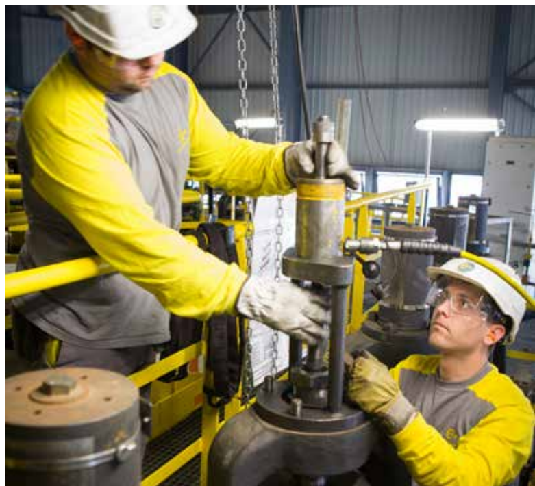
Cattenom – Work on a steam valve
