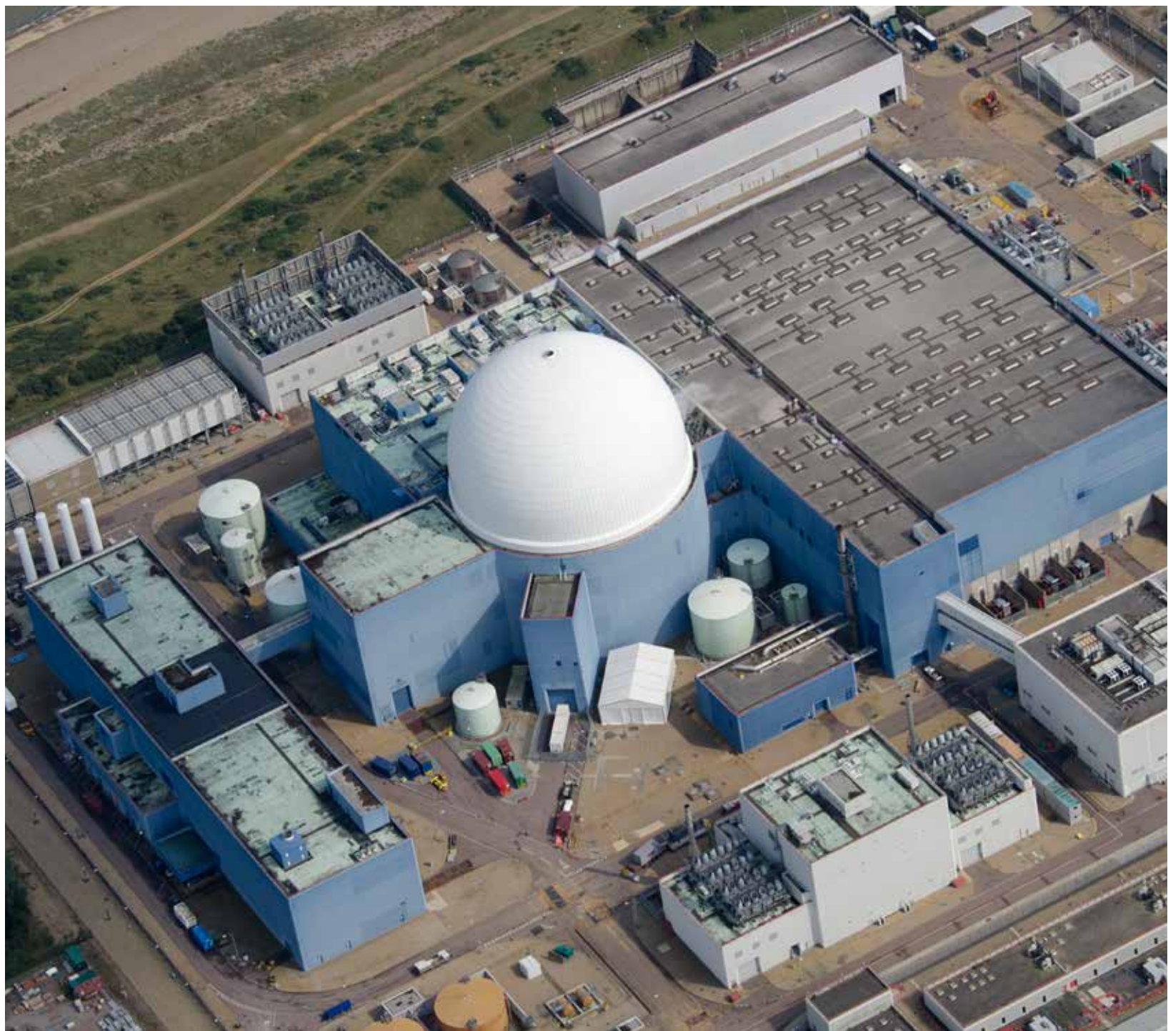
Sizewell B power station
