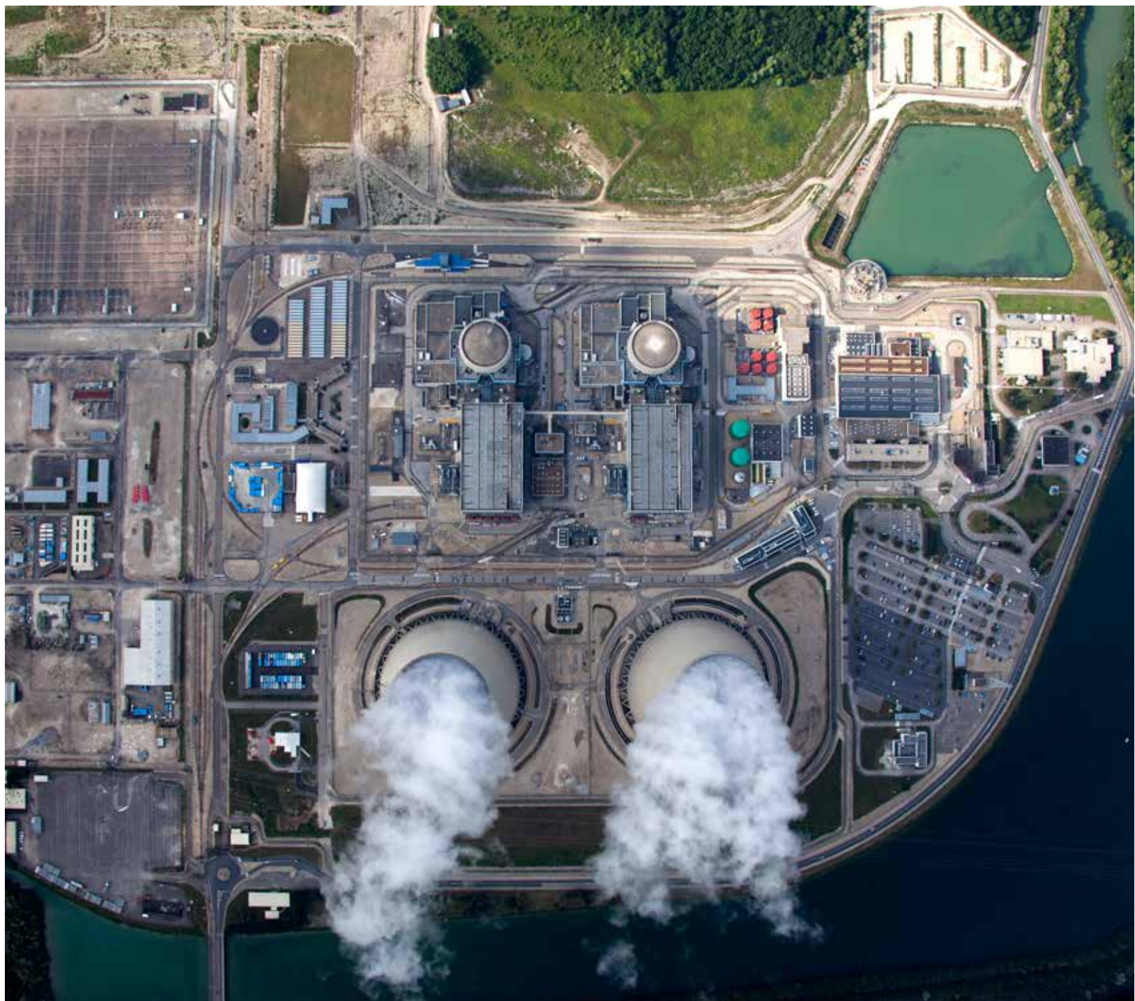
Nogent-sur-Seine power station
