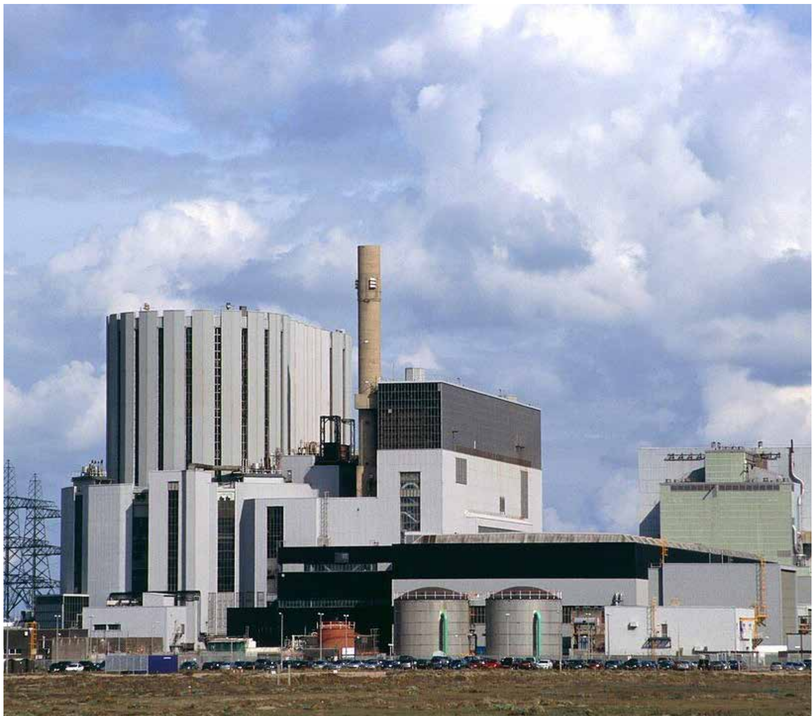
Dungeness B power station
