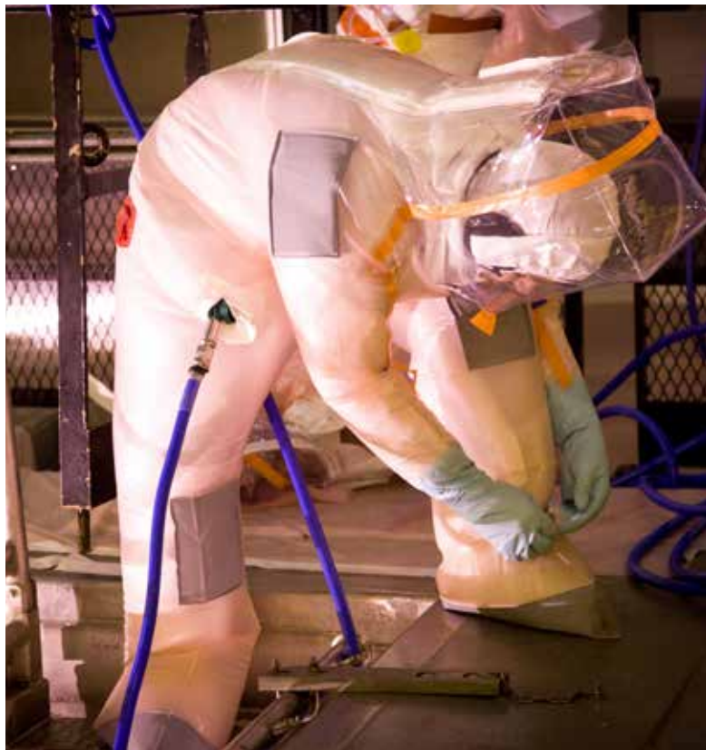
Cattenom - RCA work in ventilated airtight suit
