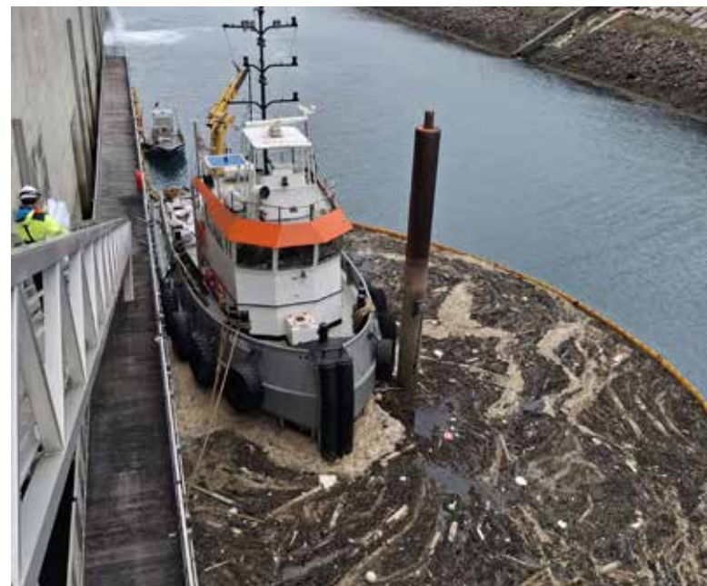
Flamanville 3 - Cleaning debris accumulated in the channel
