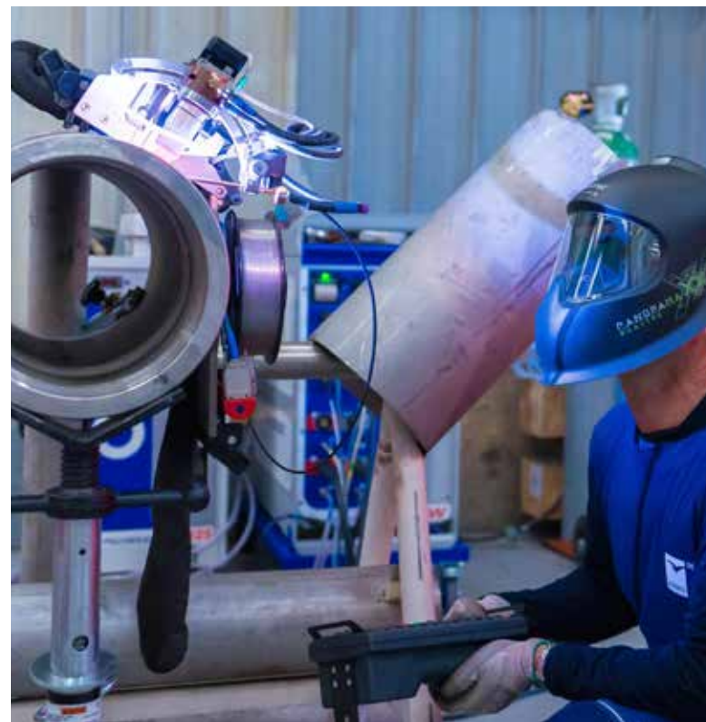
Cattenom – Automated welding during pre-fabrication work
