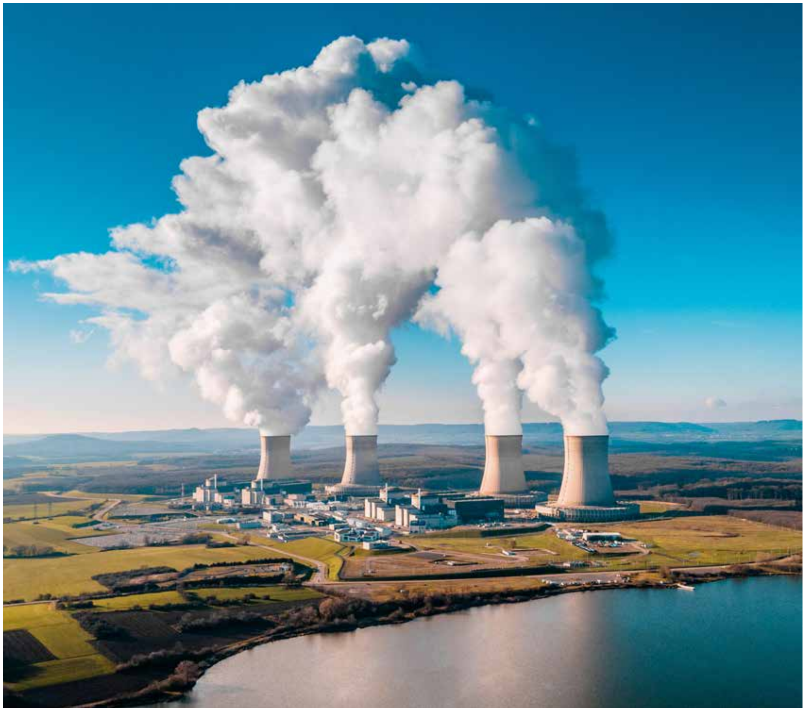
Cattenom power station
